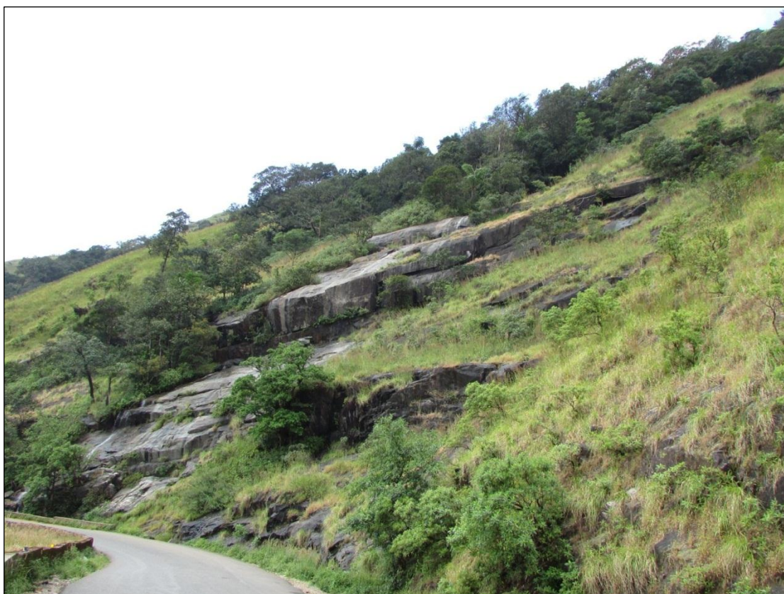
Photo – 14: Valley side dipping jointed rock (granite gneiss) exposed along Charmudi Ghat section in TS no 48O/08.
