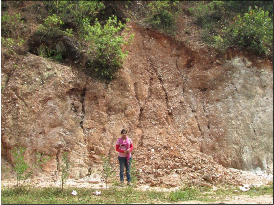
Photo – 1: Active debris slide (Slide Name: KAR/CKM/48O08/2017/001) along Kalasa – Kotighere road section in TS no 48O/08 (Latitude - 13^{\circ} 13' 22.64'' N, Longitude - 75^{\circ} 21' 59.47'' E).
