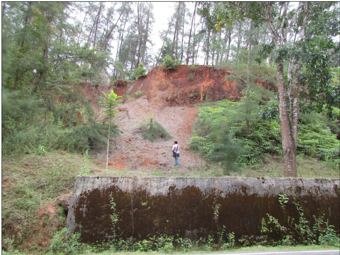
Photo – 2: Active debris slide (Slide Name: KAR/CKM/48O08/2017/013) along Kalasa – Kudremukh road section in TS no 48O/08 (Latitude - 13^{\circ} 13' 37.07'' N, Longitude - 75^{\circ} 21' 11.93'' E).
